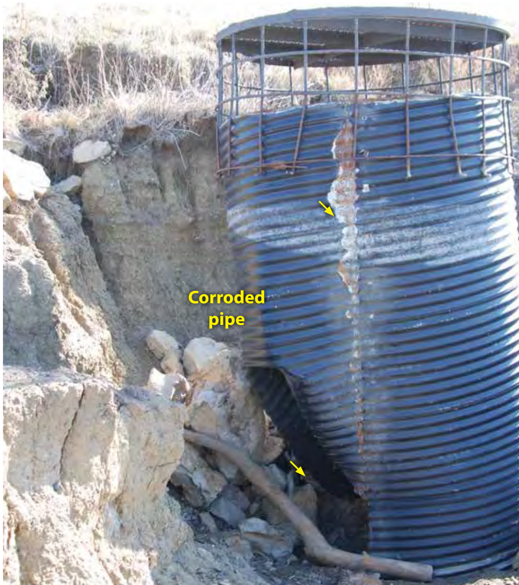
Figure 23. Cavities (or soil piping) in a dam. Piping may occur along improperly backfilled structures or from leakage through corroded metal pipes.
