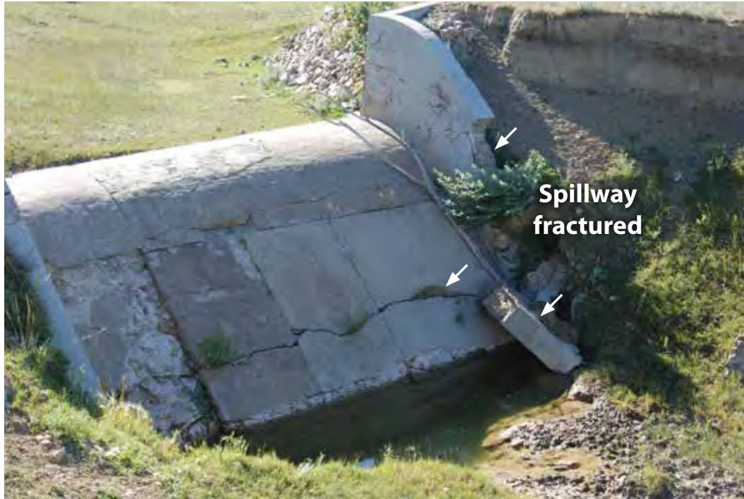
Figure 20. A cracked, slumped, and broken concrete spillway may be unstable, as discharge can access and undermine the soil and sediment beneath and adjacent to the spillway.
