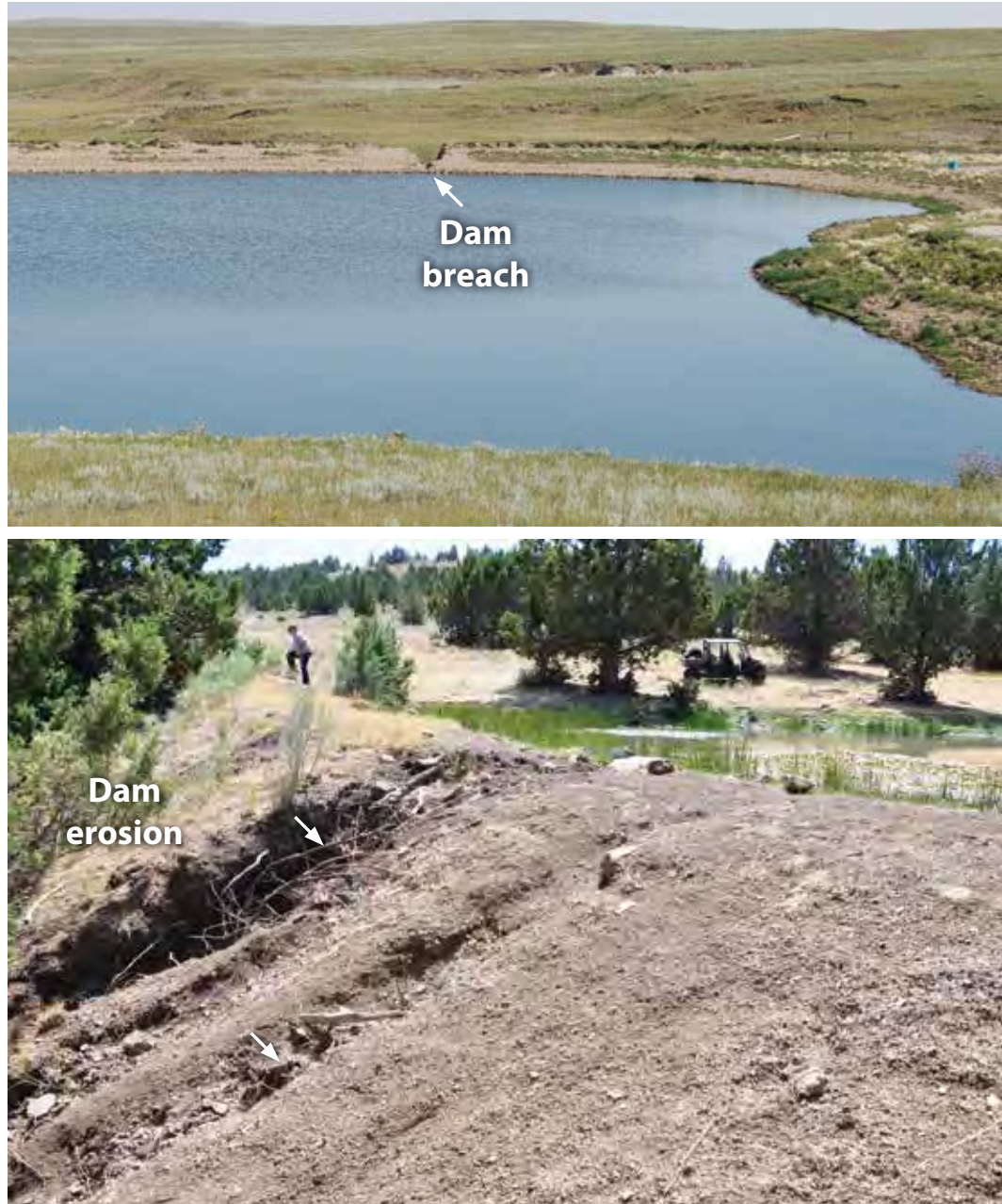
Figure 22. Water overtopping a dam can cause dangerous erosion of the dam.
