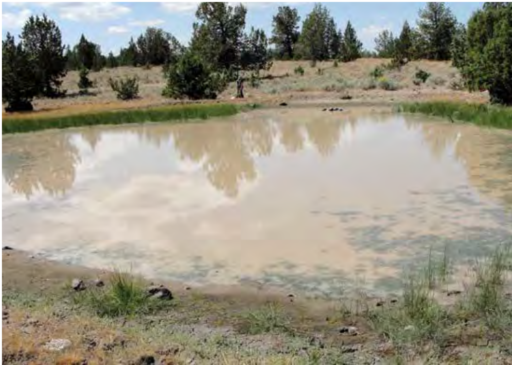
Figure 29. Shoreline not covered with an adequate amount of stabilizing riparian-wetland vegetation to protect the soil surface and dissipate energy from overland flows, and wind and wave actions, or to resist physical alteration.
