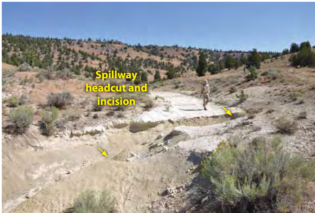
Figure 21. A 3-5 m deep headcut migrating through the spillway threatens the integrity of a dam.
