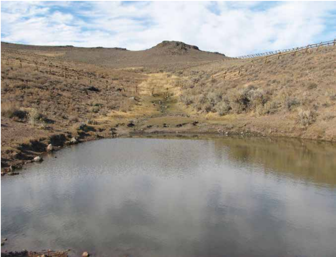
Figure D-3. Artificial stock pond constructed for livestock water. A vegetated drainageway feeds the pond and is mostly fenced. Water rights and social and economic factors likely prohibit this pond from being removed; therefore, it is relatively permanent. This structure was not intended to provide riparian-wetland values. For this site, question #1 would be answered “yes,” and PFC would not be done. However, potential would be estimated, and PFC would be completed for the vegetated drainageway. In this instance, if a PFC assessment is done on the drainageway, the pond (not assessed) may have the potential to impair the drainageway (e.g., headcut moving up into the assessed drainageway).
